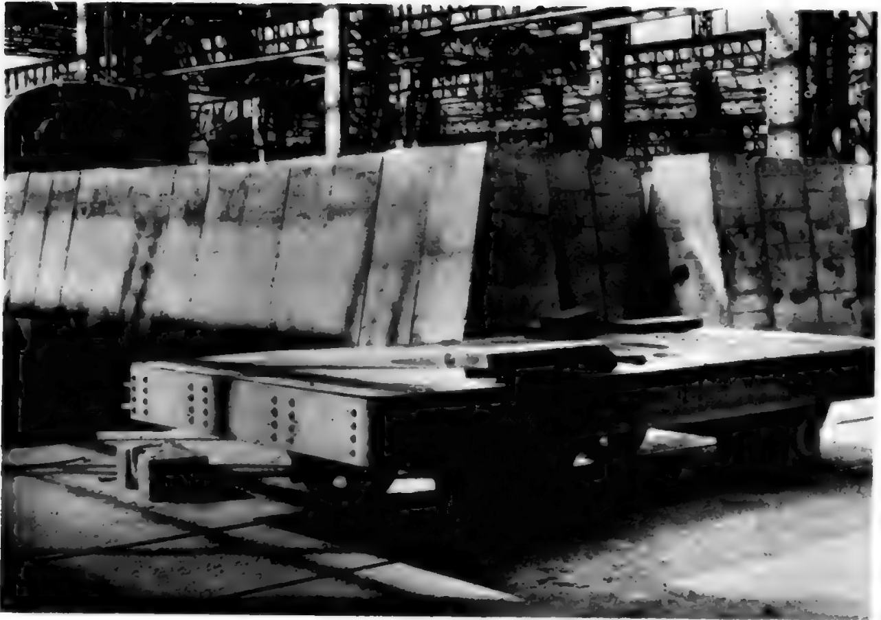
Figure 12.37a. Precast, reinforced-concrete blast walls (0.85 mile from ground zero at Nagasaki).
